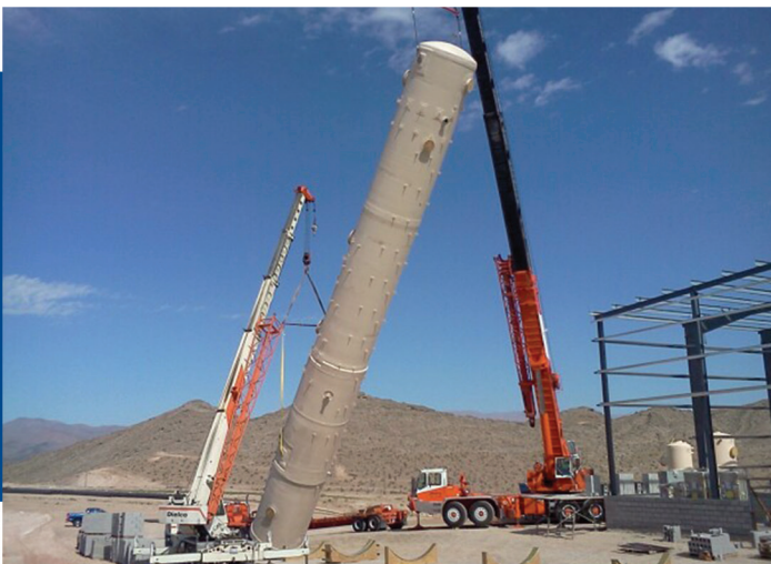
H 2 S removal via liquid phase stripping, 9' diameter x 87' OAH, skirt supported, dish bottom vessel. Furnished complete with FRP ladder system and four 90° - 180° vessel supported platforms.
